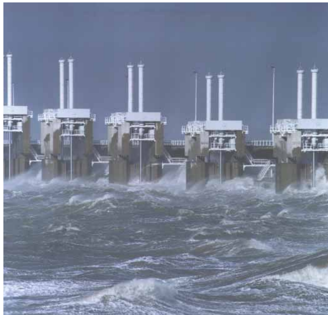
Storm surge barriers in the Netherlands, part of an extensive flood protection system built since the 1953 flooding disaster.
